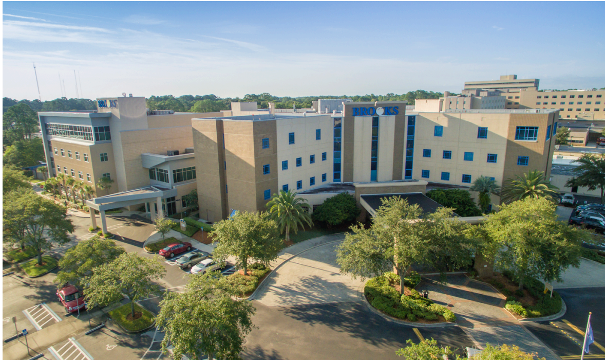
Exterior of Brooks Rehabilitation
