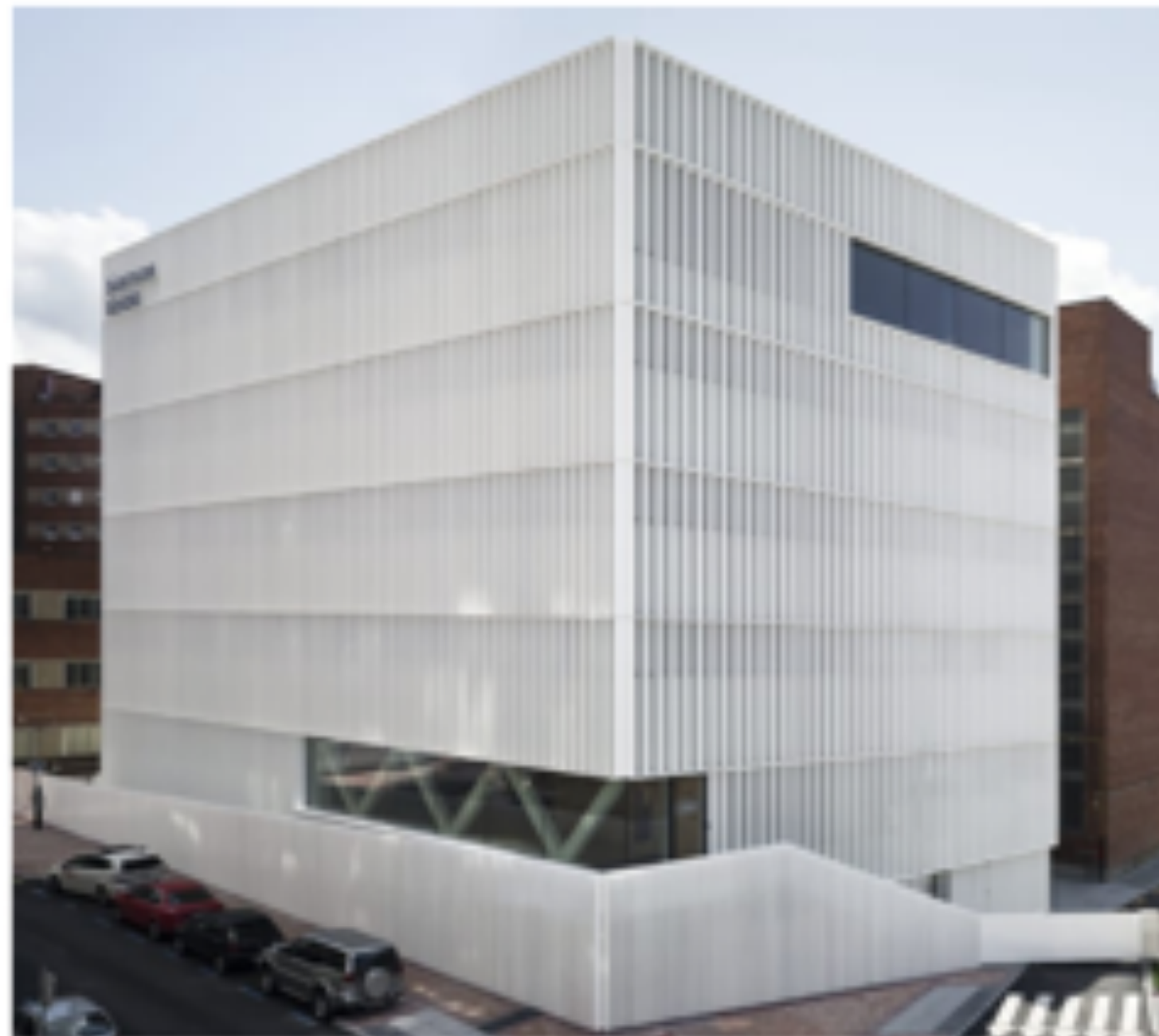
Exterior image of Cruces University Hospital (from its website)
