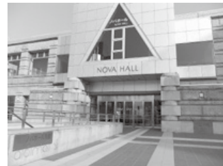
Front entrance of NOVA HALL when coming from A3 Exit
